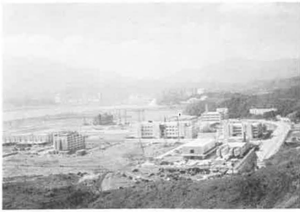
Tai Po Industrial Estate's overall view. Page 21.
